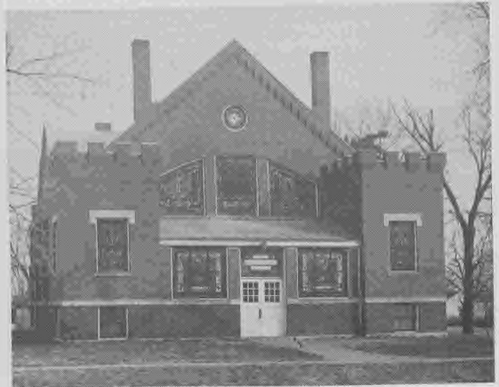
LATHROP BAPTIST CHURCH ERECTED IN 1915
