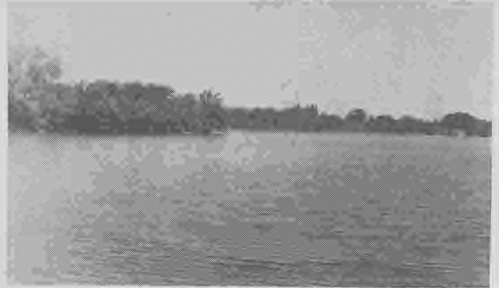
THE OLD RESERVOIR
