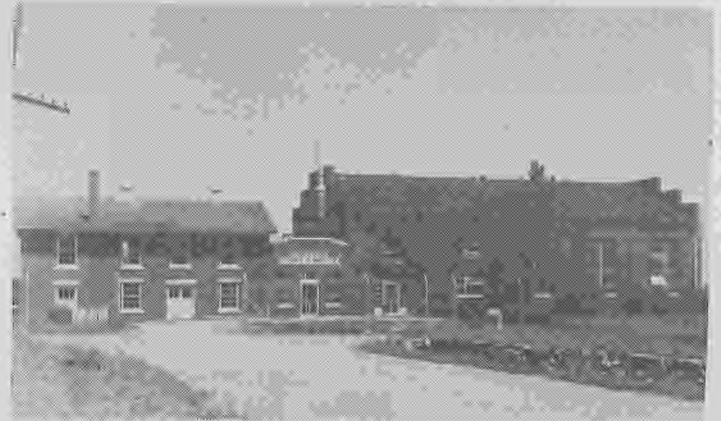
MUNICIPAL LIGHT PLANT
