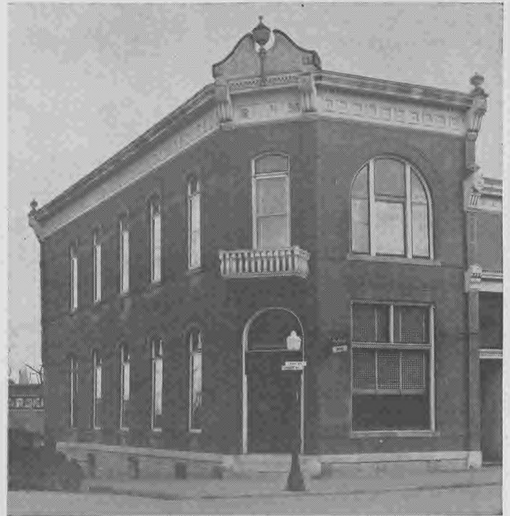
MIDDLE STATES UTILITIES OFFICE AT PLATTSBURG
