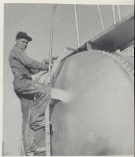
J. D. Hahn Storage Plant Hetro Gas Company
