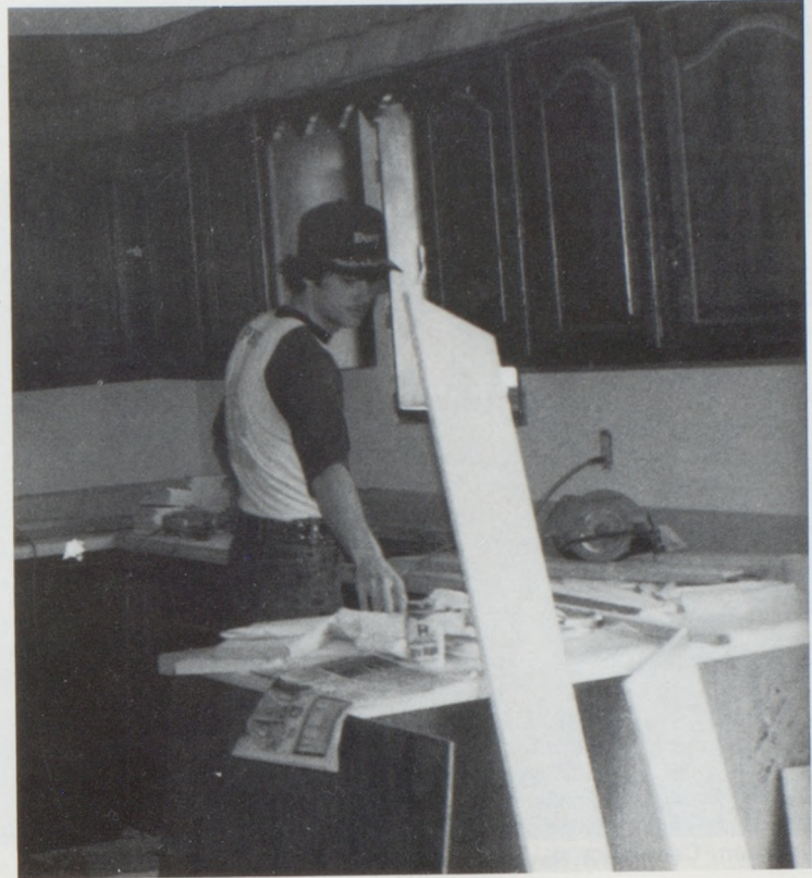
Phil Armstrong works on kitchen
