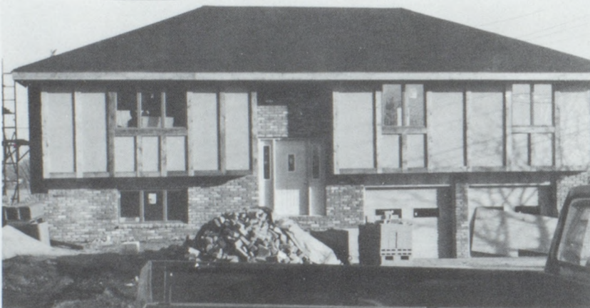
The thirteenth carpentry house before completion.
