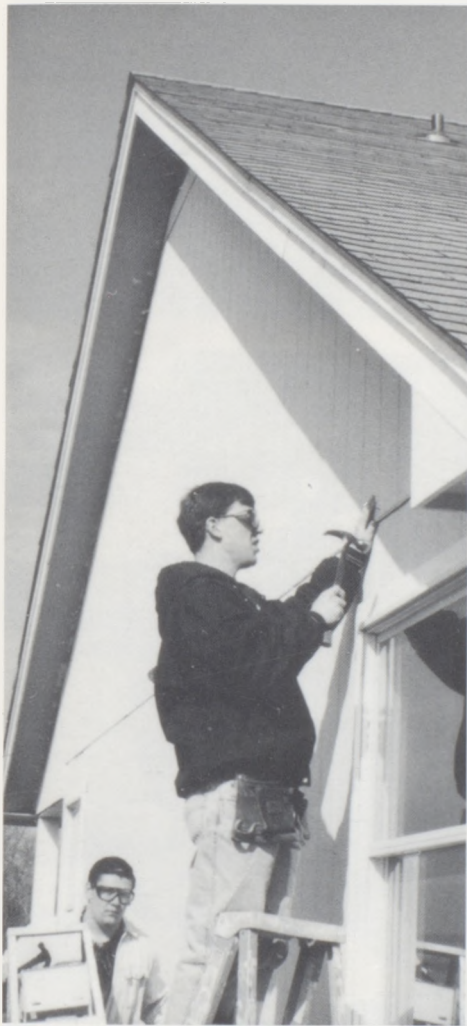
Chris Drager concentrates while hammering trim onto the carpentry house.
