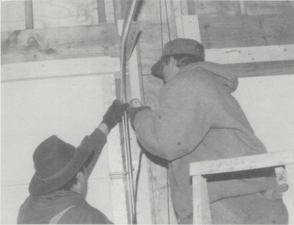
M r. Vaughn helps Joe Reickard hang the track for the garage door.
