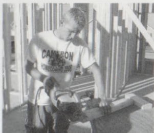
Tyler Oitker cutting boards for the rafters.
