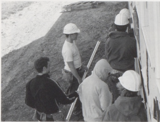
The crew works together to finish the siding installation.
